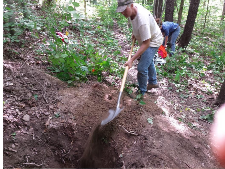
Locating and Verifying Unmarked Legacy Wells
